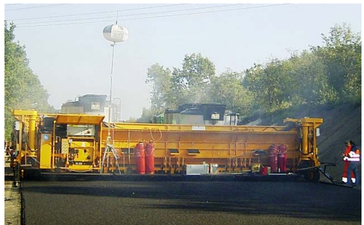
Gussasphalt (mastic asphalt) - finisher with Powermoon-site lighting
