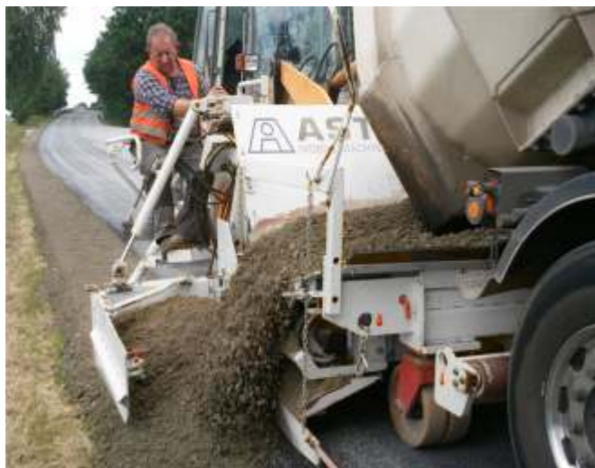
rapid material placing with flow control
