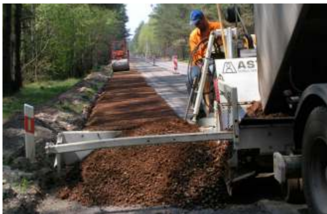
Road extension with 2m working width - capacity for 400 to per hour
