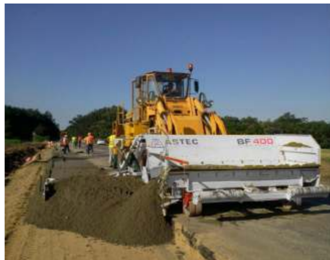
road extension with 2m working width
